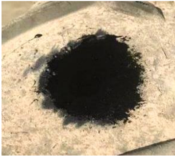
Hole and rip repair
