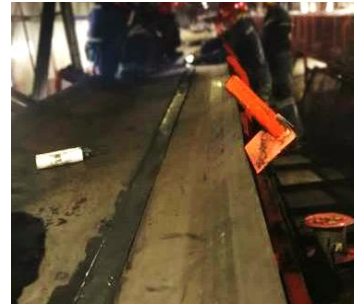
Long rip repair
