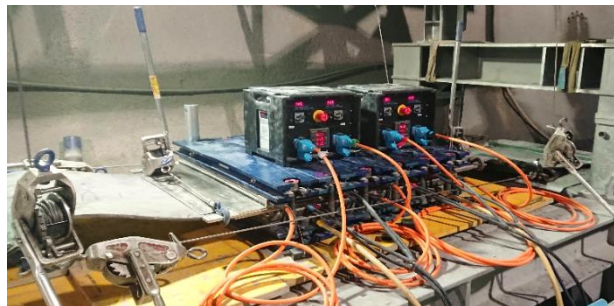
Steel cord belt splicing
